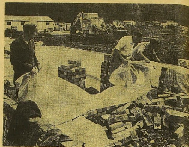
Work has begun on new homes at Griffin Close.
