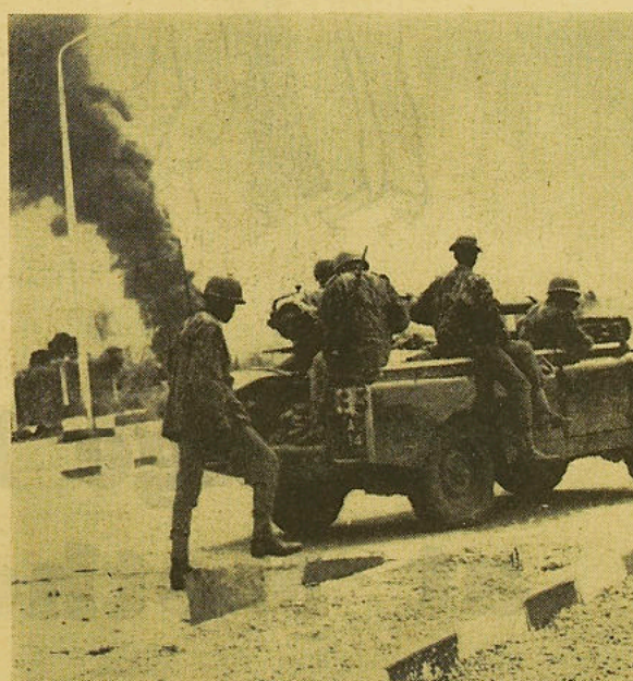
Smoke billows skyward from burning oil tanks in Onitsha (background) across the Niger River at Asaba approach to the damaged bridge seized by Federal forces.
