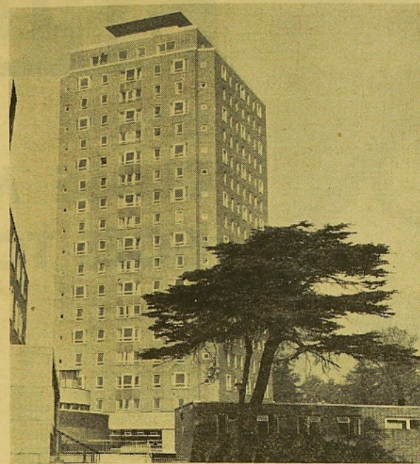
HIGH HALL, WHERE RESIDENTS ABOVE THE TENTH FLOOR HAVE NO COLD WATER BETWEEN SEVEN AND NINE O'CLOCK IN THE MORNING.
