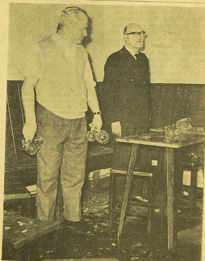
Staff clearing up some of the debris after the bar had been closed.
